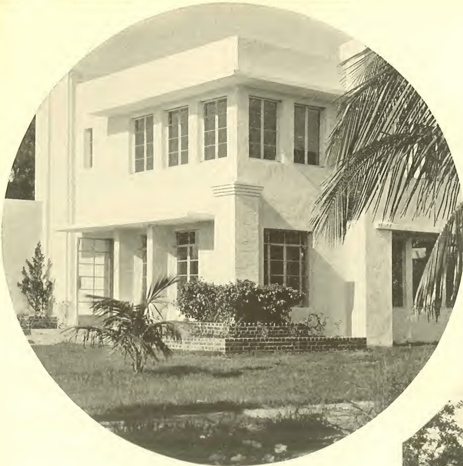
One of the scores of new concrete homes built or under construction at Miami Beach, Fla., this gracefully modern house has concrete masonry walls with portland cement stucco finish. Its cost—$6,000. Its architect—H. E. Collins, Miami, Fla.
